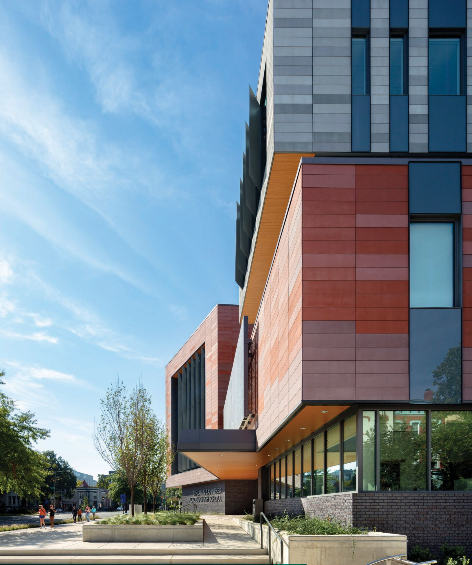
BENJAMIN BANNEKER ACADEMIC HIGH SCHOOL, WASHINGTON, DC | FIRST HIGH SCHOOL IN THE DISTRICT TARGETING NET ZERO ENERGY
